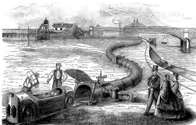
The first full-scale trial of Rammell's pneumatic despatch was at Battersea Fields during the summer of 1861. A single tube was installed, 452 yards long, with curves of up to 300 feet radius and gradients of up to 1 in 22.2 ft., narrow gauge track was laid inside the tube. Wheeled capsules were fitted with vulcanised rubber flaps to make an air seal. Power was provided by a 30 horse-power steam engine with a 21 feet diameter fan. Single capsules weighed up to 3 tonnes, and achieved speeds up to 40 mph.
